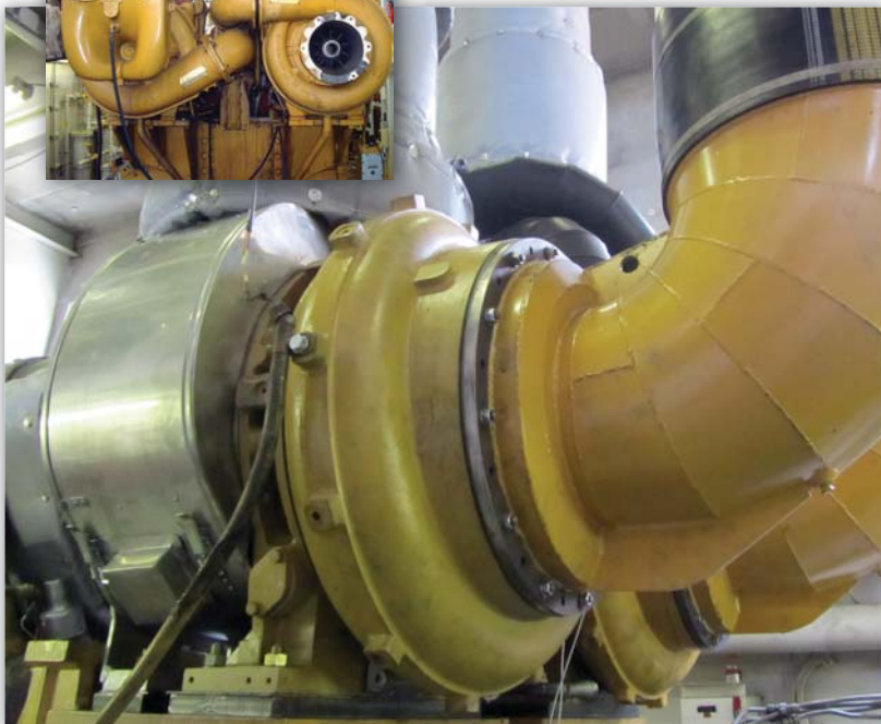
After: Napier NA297 turbocharger installed with new platform and air intake.
